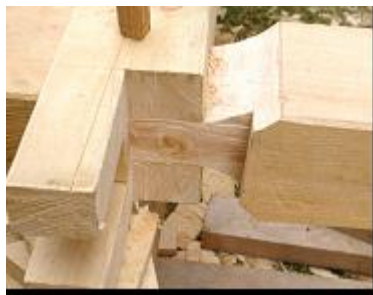
The joint used in Grindbygningen between the stav and the bete which form the grind.
