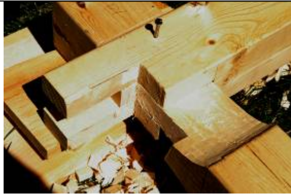
The stavoyre, the joint between the stav and the bete.
