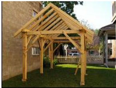
The completed Grindbygningen ready for the roof and sides.
