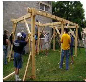
The stavlaegje supports the sperre, the rafters, in a series of grooves so that no nails are needed to fasten the sperre to the stavlaegje.
