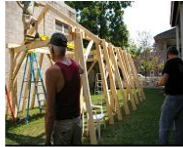
Next we installed the sperre, or rafters
