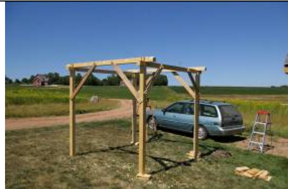
The grinds set upright with the stavlaegjer in place. My grindbygningen has only one section, and the height is slightly too tall to match Viking proportions since my betes were limited to 8' without a special order, which would take 3 weeks.
