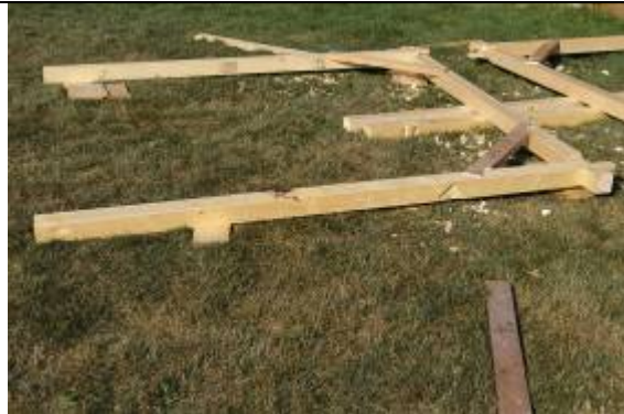
The completed grind. The skraband or braces were made out of scrap 2x4. I am using temporary pegs made from pine, but I will have to change to something tougher.
