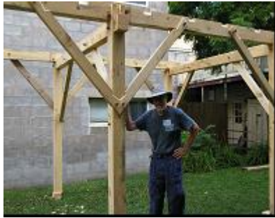
The braces, skraband, used a dove tail joint construction.
