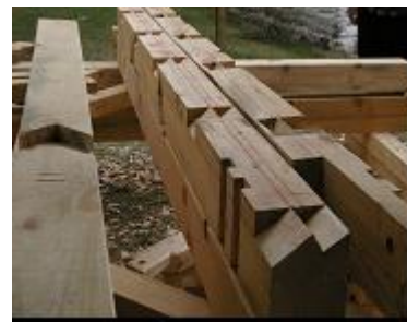
The stavlaegje supports the sperre, the rafters, in a series of grooves so that no nails are needed to fasten the sperre to the stavlaegje.
